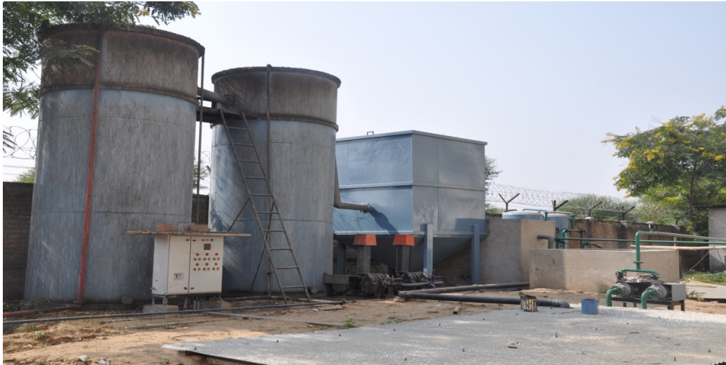
Fig 1, Sewage Treatment Plant At Ces, Jaipur
